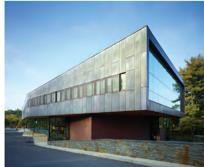
The JOHN W. OLVER TRANSIT CENTER in Greenfield MA Building: Charles Rose Architects Photography: John Linden
