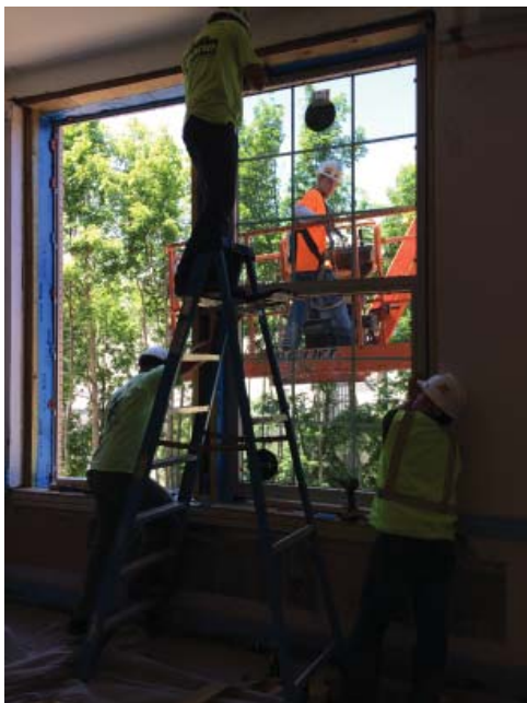
Chandler Architectural Products setting up a full size window mock up at the Conte School
