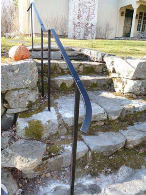
Historic Handrail Photo: John Graney
