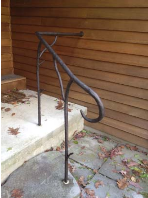
Branch Handrail Photo: Laurel Graney
