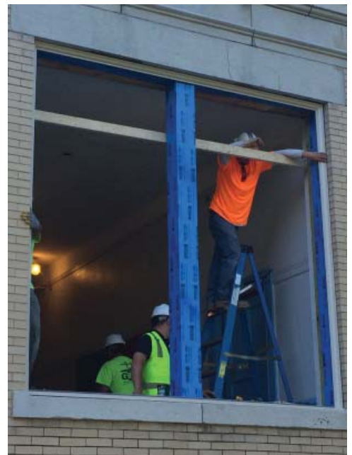
Chandler Architectural Products setting up a full size window mock up at the Conte School
