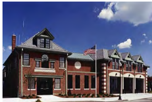
Milford Fire Department
