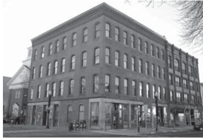
Main Street's Arts Block (1876) renovation design by Margo Jones Architect
