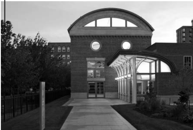
Stephen Jablonski Architects Lymann & Merrie Wood Museum of Springfield History Springfield, MA photo: Michael Janeczek
