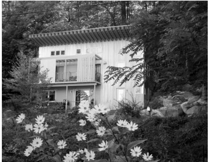
Stephen Gerard Dietemann RA Anderson Residence – New Construction Great Barrington, MA photo: Ignacio Salas-Humara
