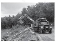
be weighed. Wall stone is sold by weight (a typical dump truck full is 20 tons).
