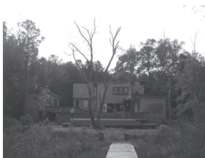
maritime woodland and expansive coastal landscape breaks the program into three structures united by a terrace and pool.
